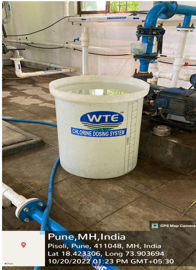
Chlorine dosing system in STP
