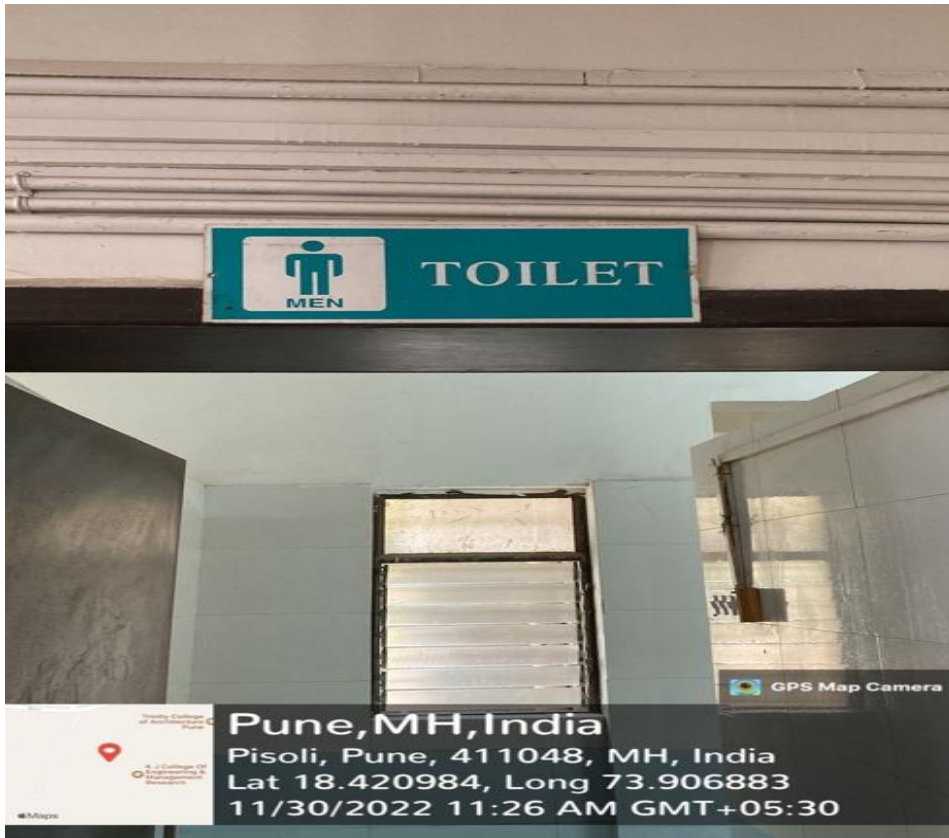
Identification signage board of male toilet
