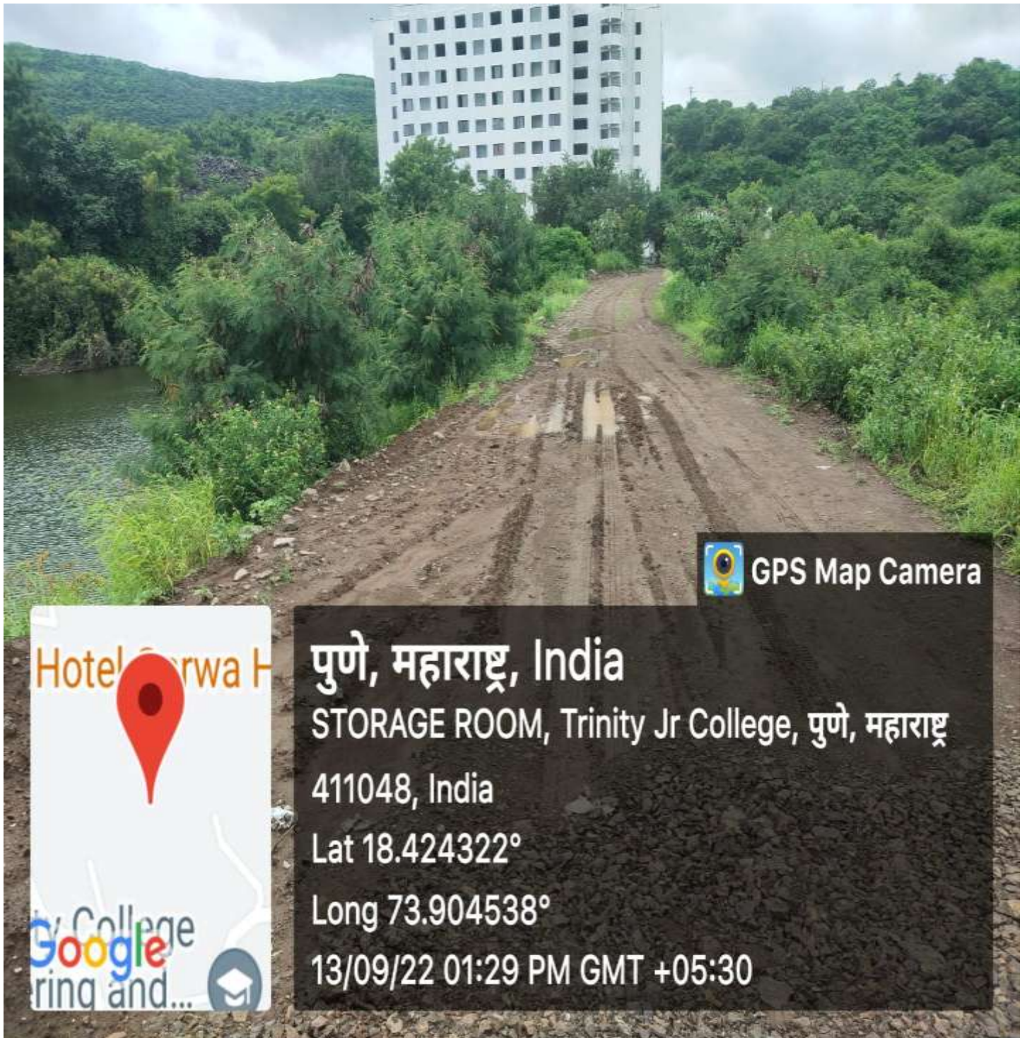
Earthen bunds constructed to create the water bodies
