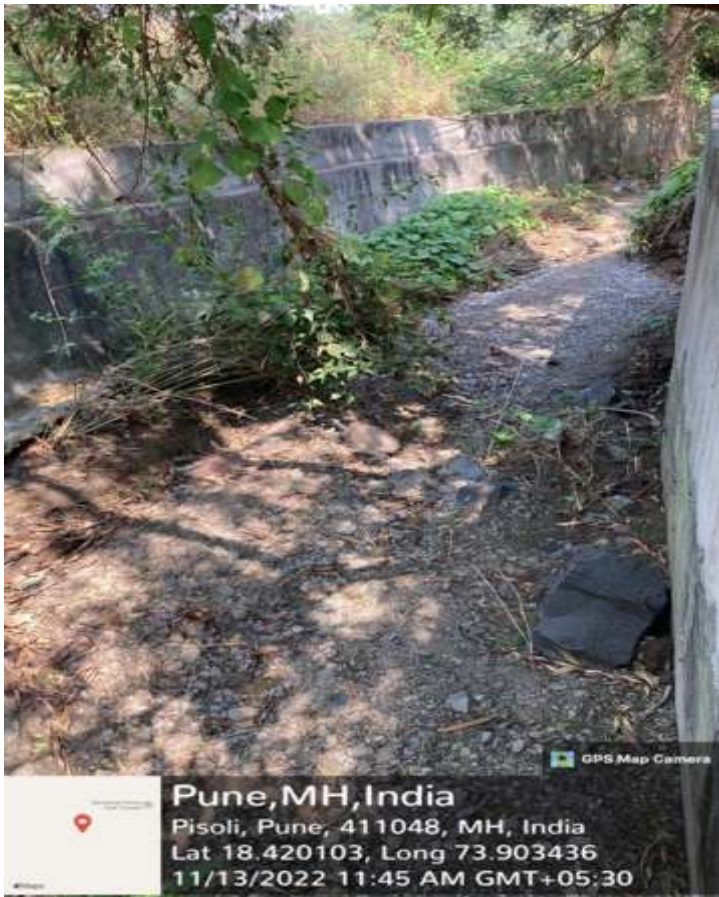
RCC channels to collect and transfer the rain/storm water
