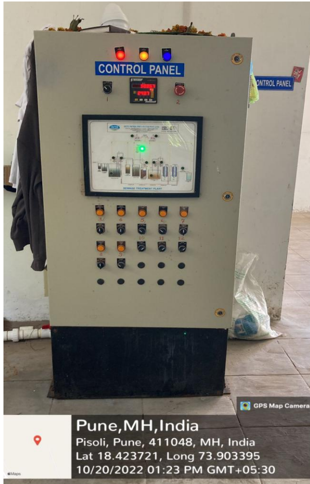
Control Panel of STP
