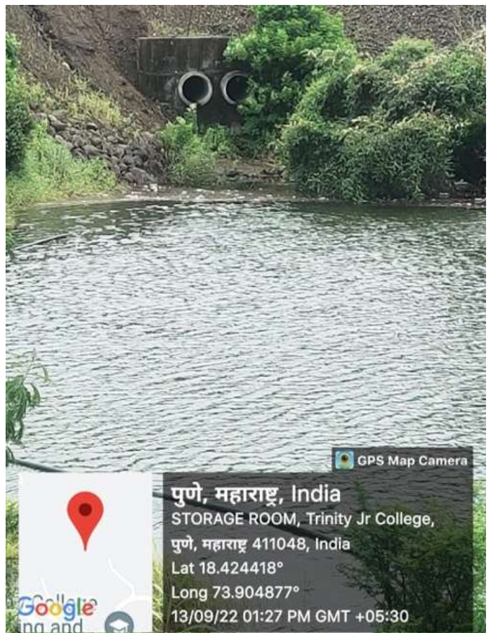
RCC pipe to collect and transfer the rain/storm water
