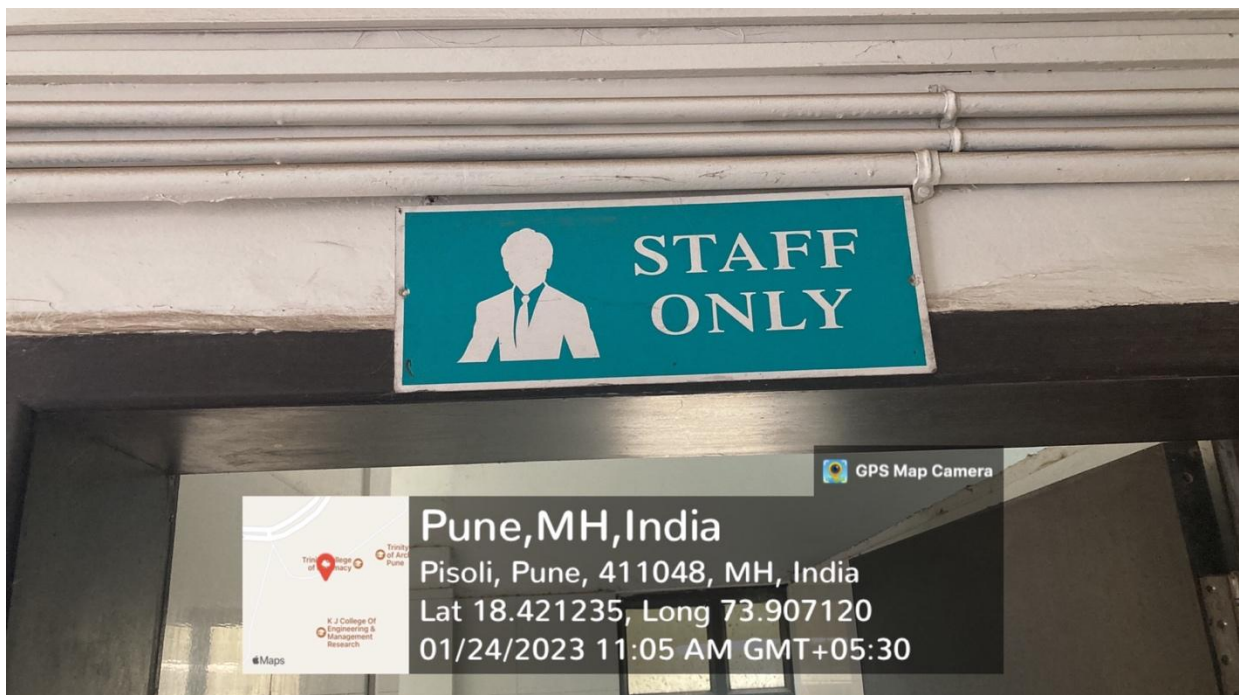
Identification signage board of male staff toilet
