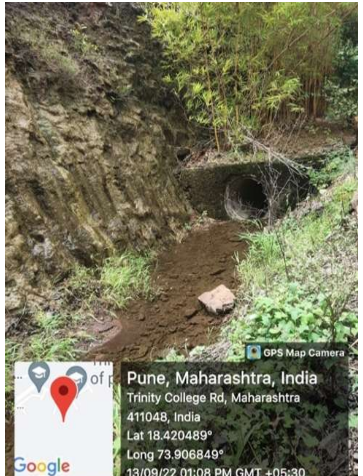
Channels to collect and transfer the rain/storm water
