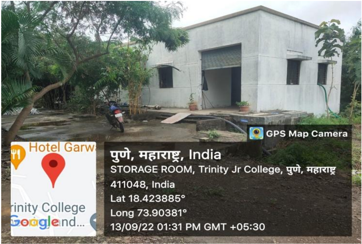
Sewage Treatment Plant (STP)
