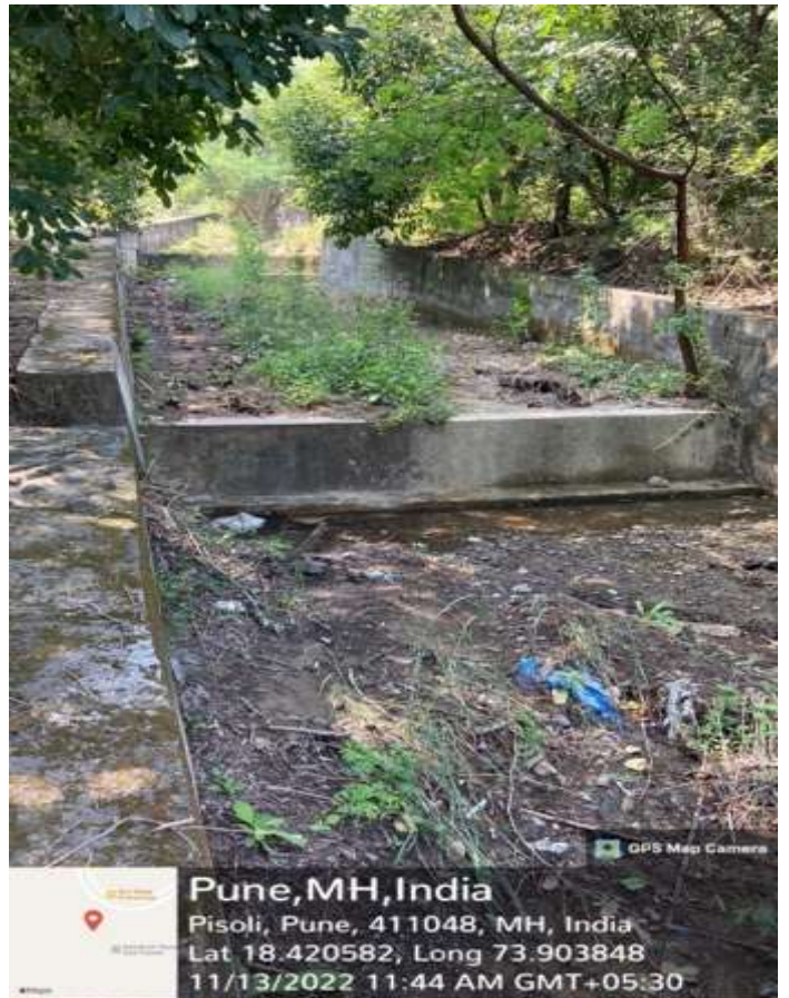
RCC channels to collect and transfer the rain/storm water
